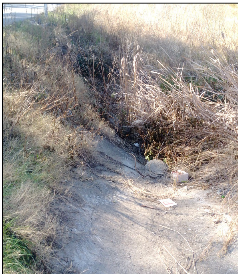
Figure 6 - Existing swale and concrete dish drain in John Renshaw Drive.
