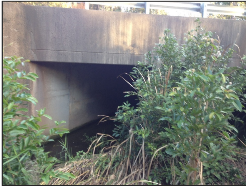
Figure 3 – Rectangular box culvert beneath John Renshaw Drive.
